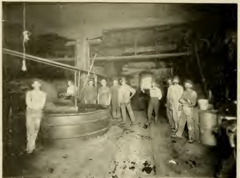
INTERIOR VIEW OF BEATER ROOM
